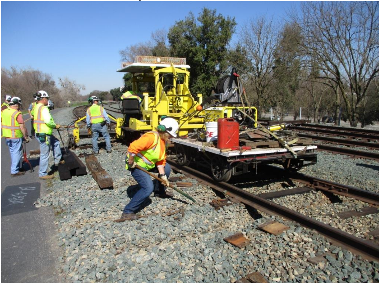
Bev digs debris out from an empty tie-crib
