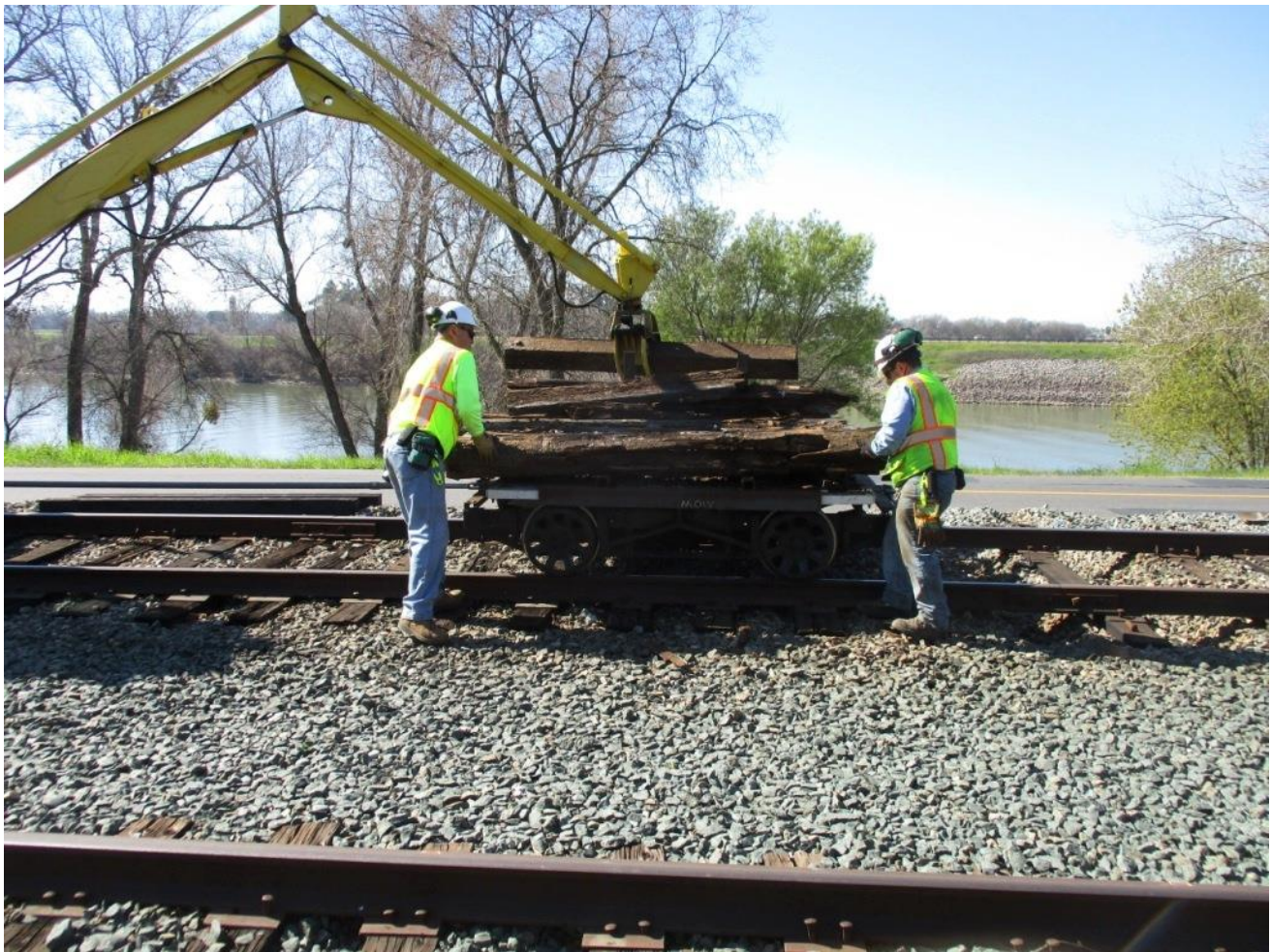
Taka and Joe adjust the load of dead-ties on the flatcar
