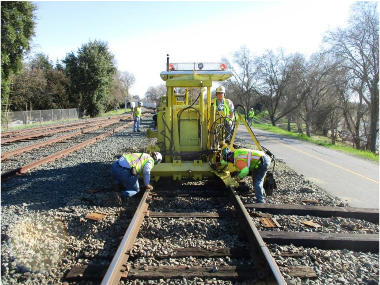
Chris C. on the 125 jacks-up the rails so that Heather and Joe can insert tie-plates
