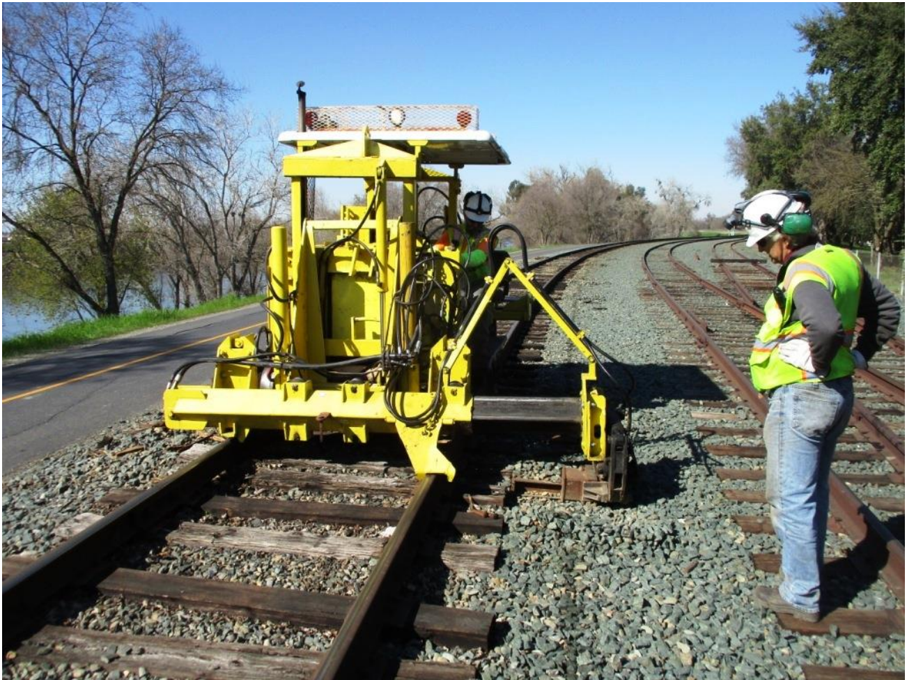
The shoving-ram is used to push out those ties that broke apart when the attempt was made to pull them
