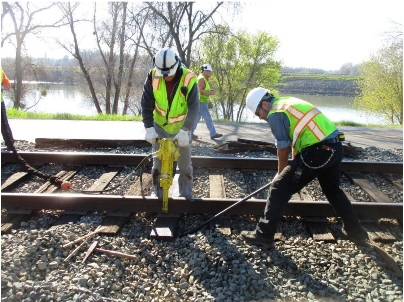
Kyle nips-up the tie as Steve drives spikes
