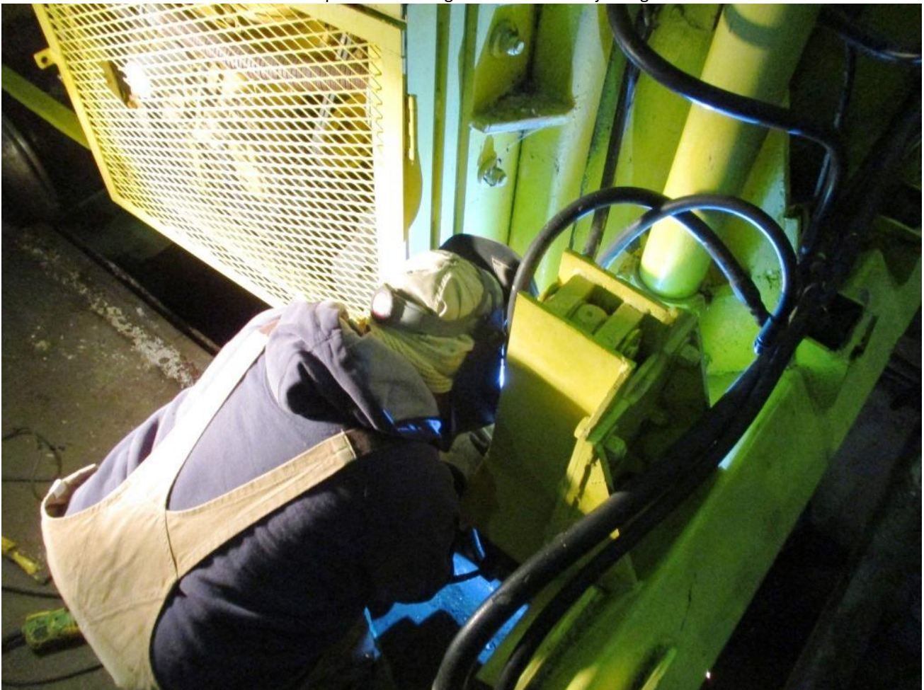
Cliff welds the securing system on the 125's jacking-ram
