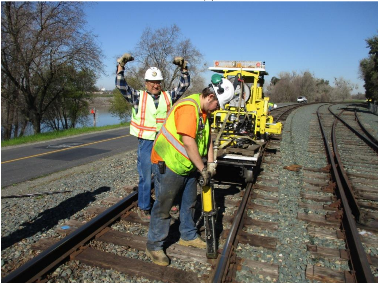
Chris C. pulls a spike with the hydraulic spike-puller as John demonstrates his famous, "I am Batman!" stance
