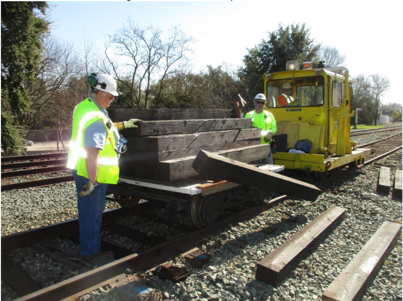
Chris C. and Taka drop new ties from the new tie bundle
