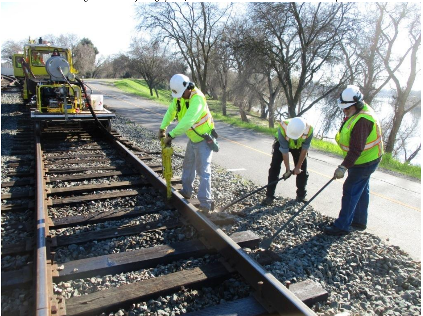
Taka drives spikes with the hydraulic spike driver as Kyle and Art nip-up the ties
