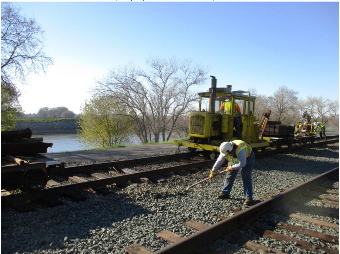
Heather uses a shovel to move ballast around and fill in any holes
