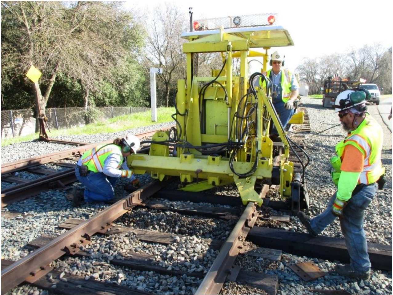
Using the 125's rail jacking system, Chris C. lifts the rail as Heather inserts a tie plate
