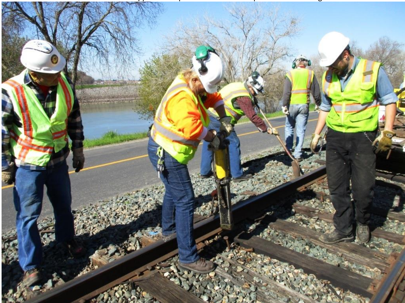
Bev pulls spikes with the hydraulic spike-puller
