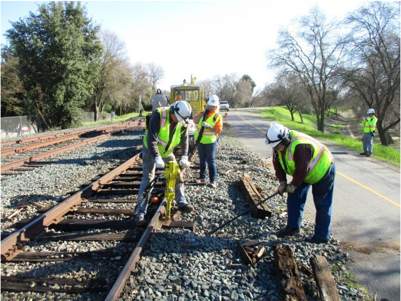
Bev monitors the hydraulic lines as Steve drives spikes and Art nips-up the tie
