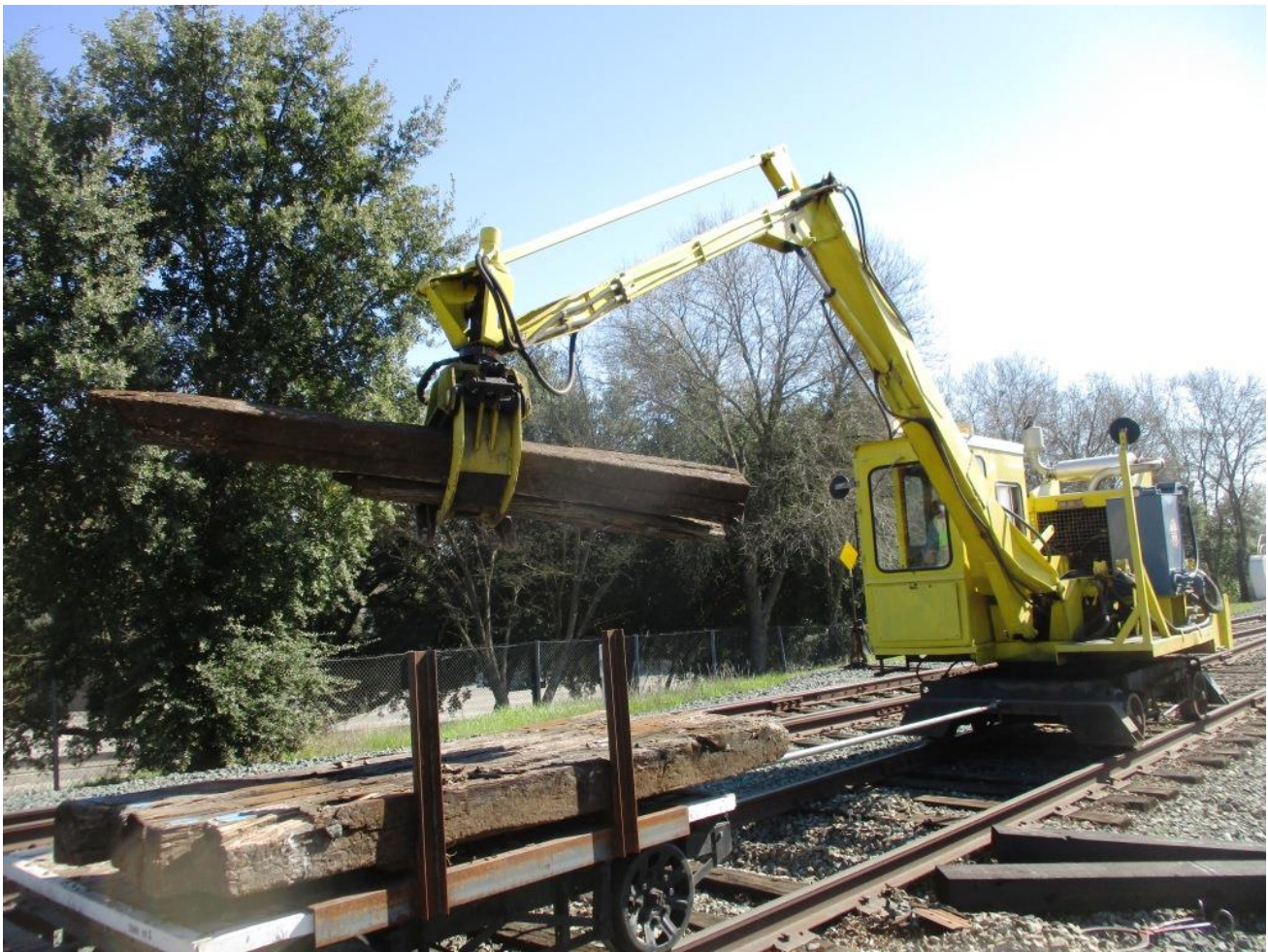
Alan brings in the tie-crane to remove the dead ties
