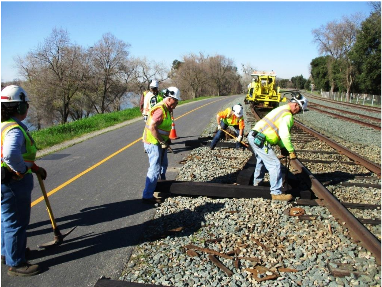
...Then place it under the base of the rail where the 125 can grab it and pull it in
