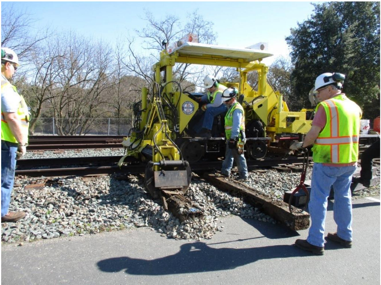
Heather does a great job pulling ties with the 125
