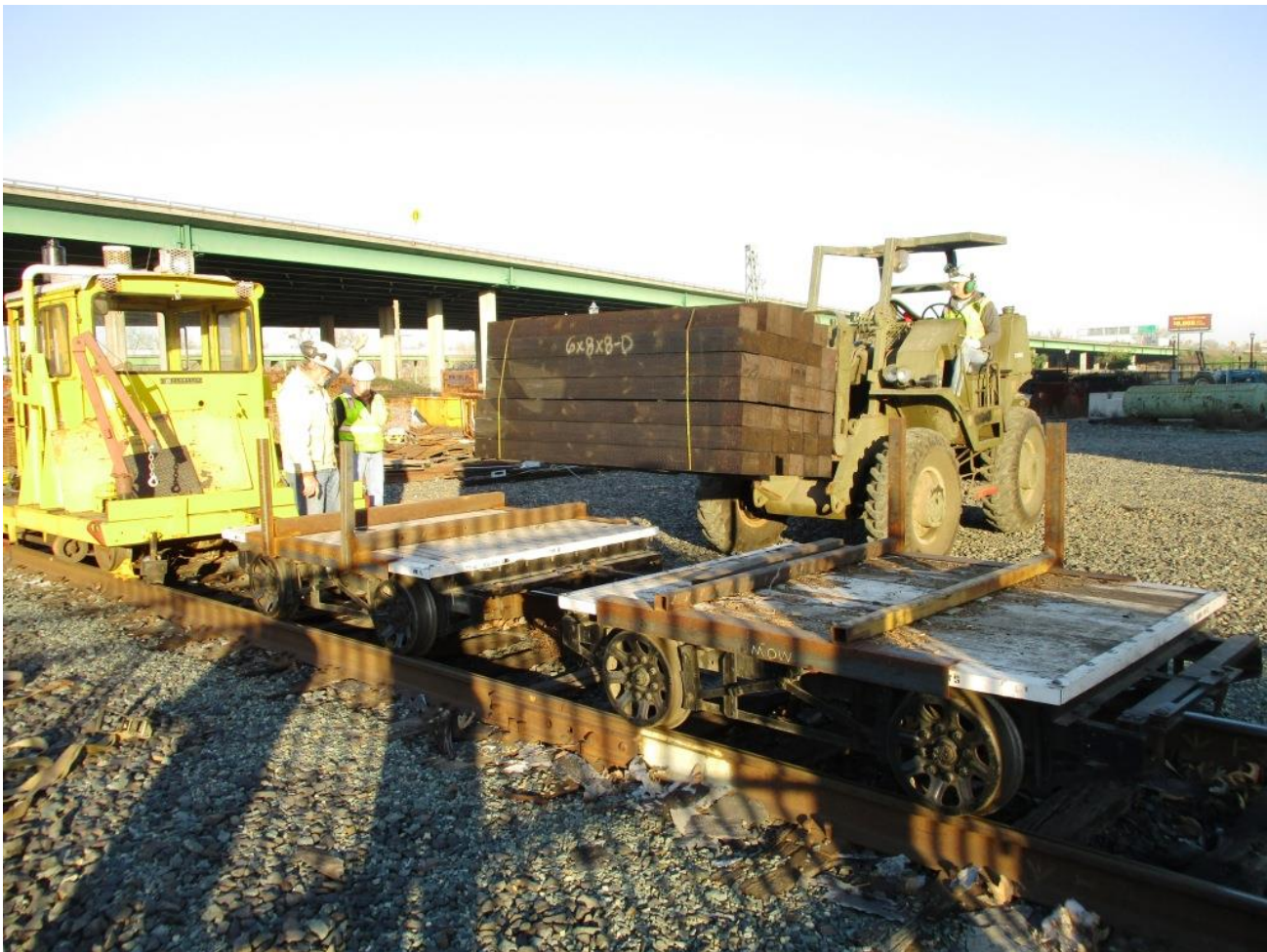
Steve on GM2 loads a bundle of ties onto a flatcar with Alan and Bill guiding
